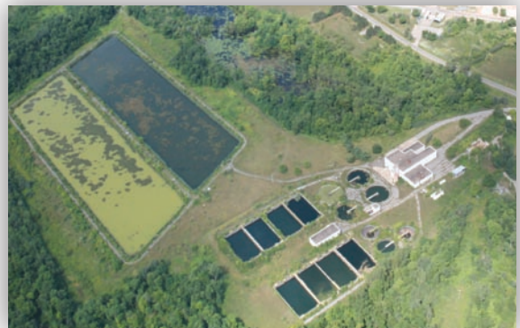
On-site wastewater treatment plant with capacity for up to 10,000,000 gallons per day, including 65,000 pounds of BODs and 30,000 pounds of primary solids
