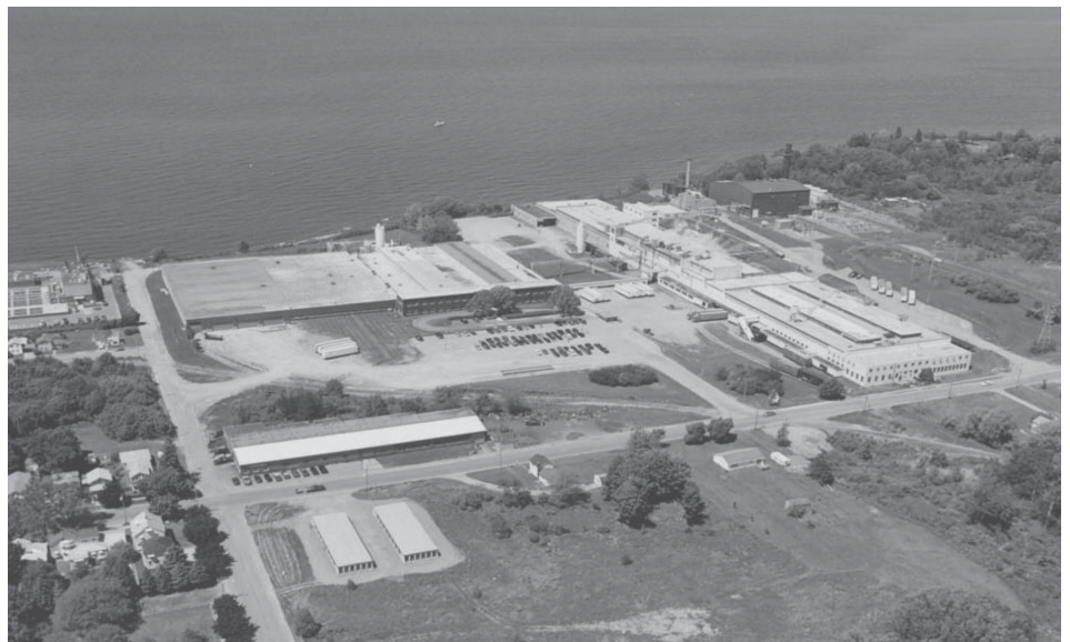
Former International Paper facility located on Mitchell Street in Oswego.
