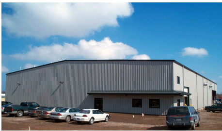
Empire Fresh-Cuts' new onion processing plant in the town of Oswego.
